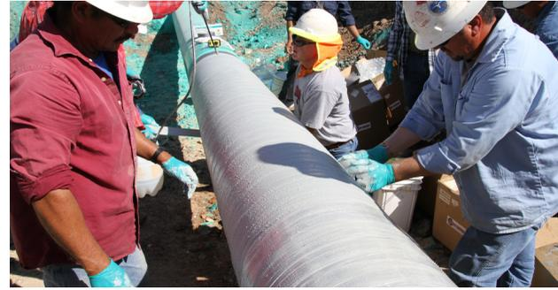
**The A+ Wrap™ System** is a high-strength, water-activated fiberglass composite pre-impregnated with moisture cured polyurethane resin. It is designed for simplification of installation for restoring the structural strength of degraded pipe with varying geometries. It is also able to be used for pressure containment under certain circumstances.
